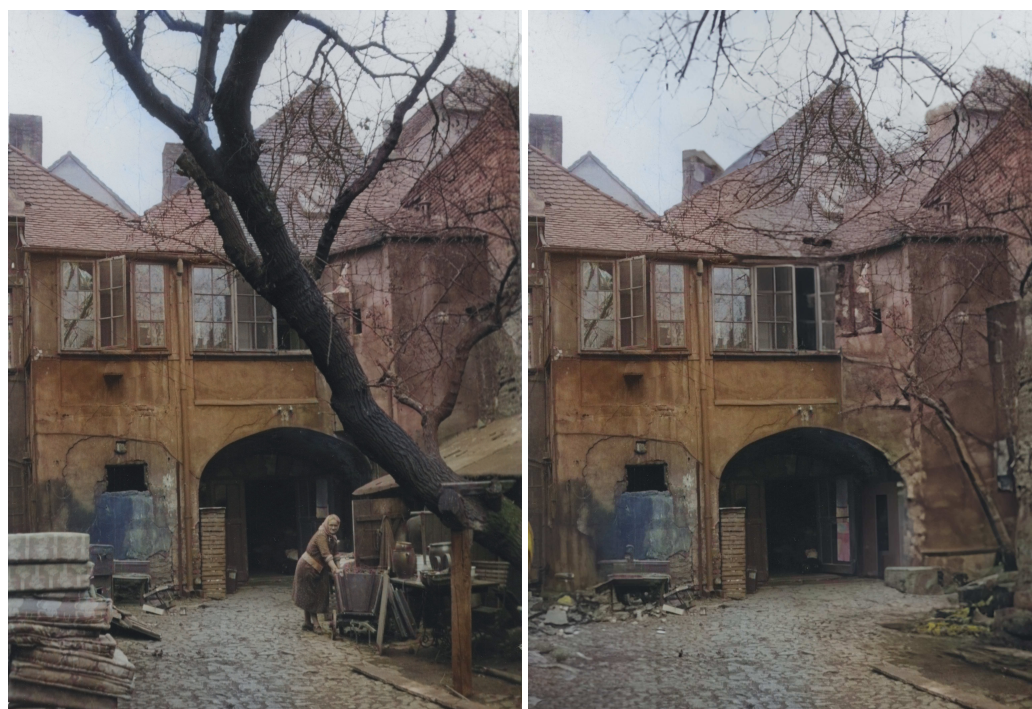
Figure 3. (Left): A sample photo where shading obscures much of the building, making reconstruction difficult. The appearance of a large part of the building is unknown and cannot be obtained even from historical photographs; (Right): Objects removed and replaced with one of the possible reconstructions of the obscured content.
